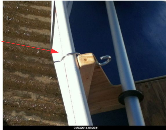
Clamp secured over the pipe
