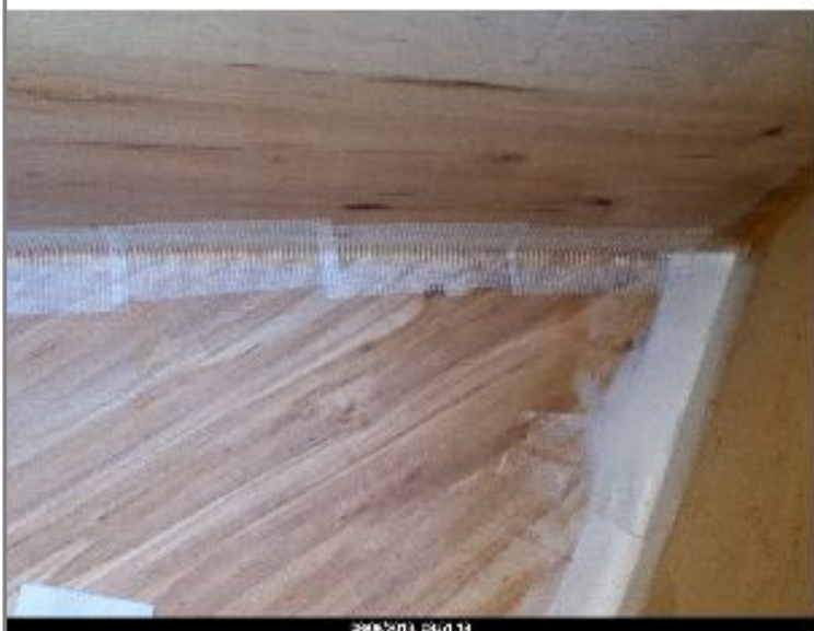
Overlapping Taped Sections
