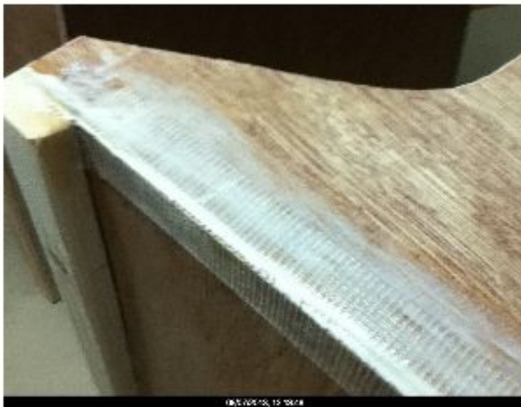
Finished taped edge
