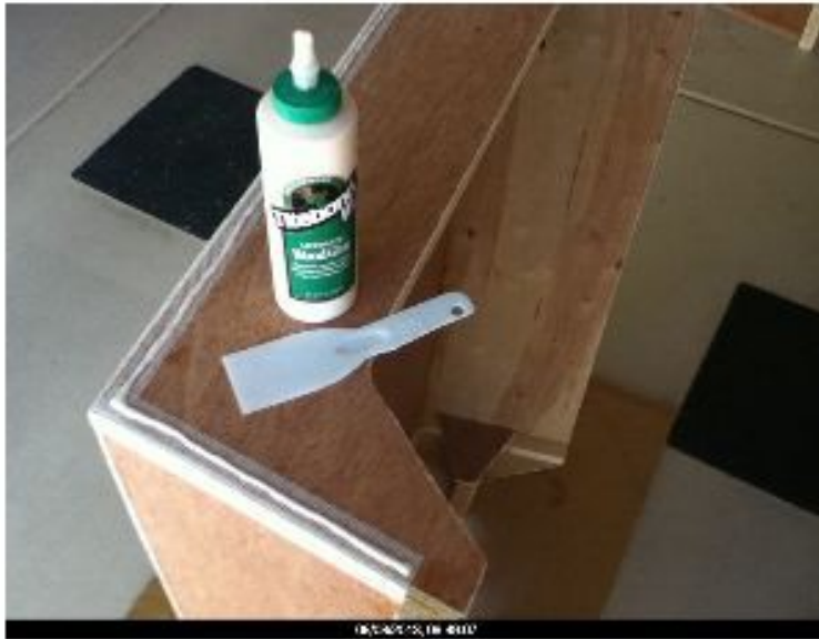
Typical glue bead size
