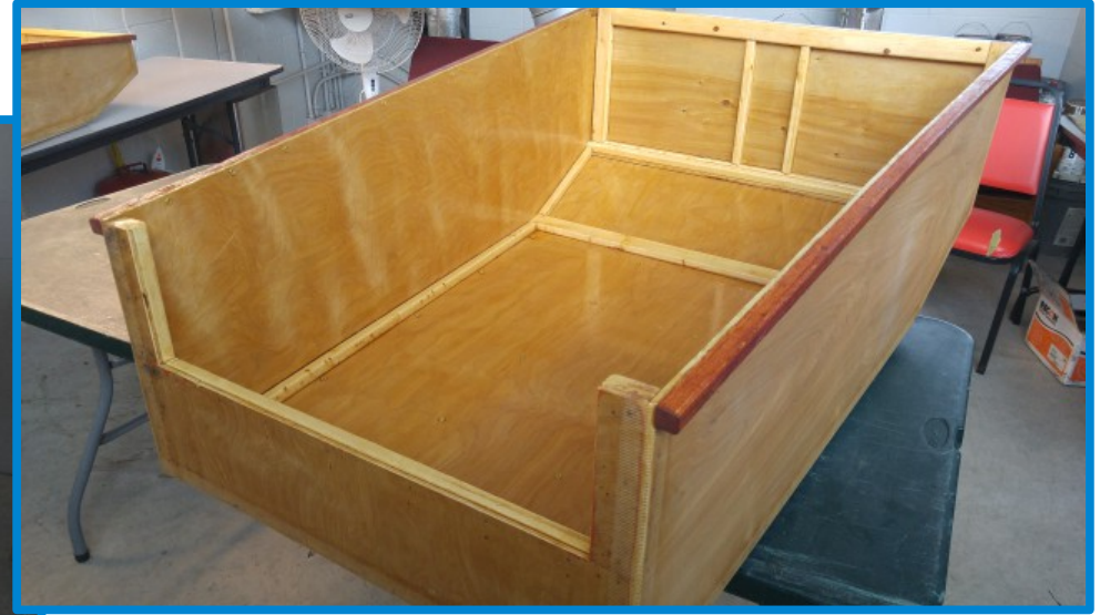
Typical inside construction of the rear module.
