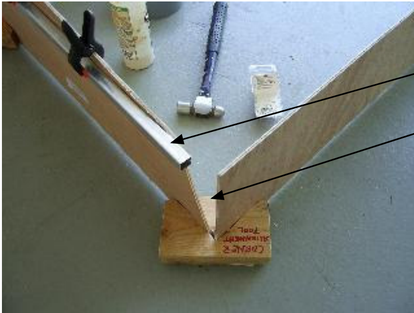
Start of Panel construction with Corner Alignment Tool
