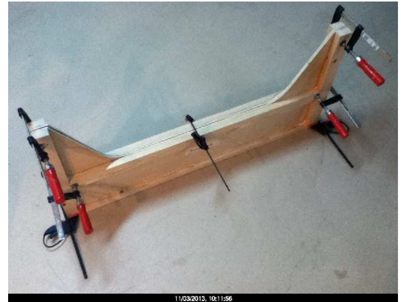
Two bulkheads clamped together to insure they mate properly. Adjust as necessary..
