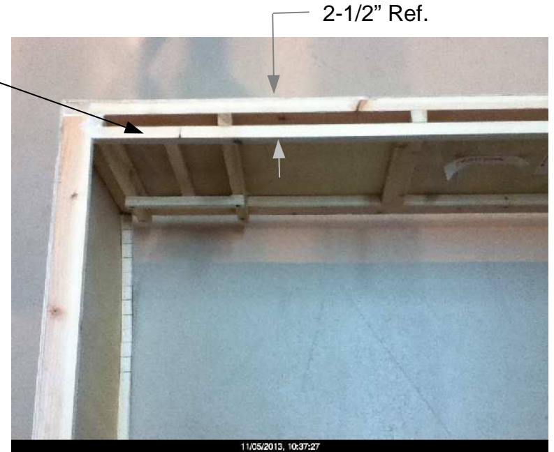
Completion of rear deck support, 1 x 1 stringer
