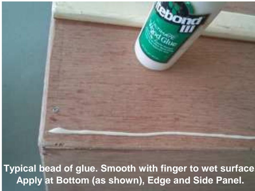
Typical bead of glue. Smooth with finger to wet surface.
