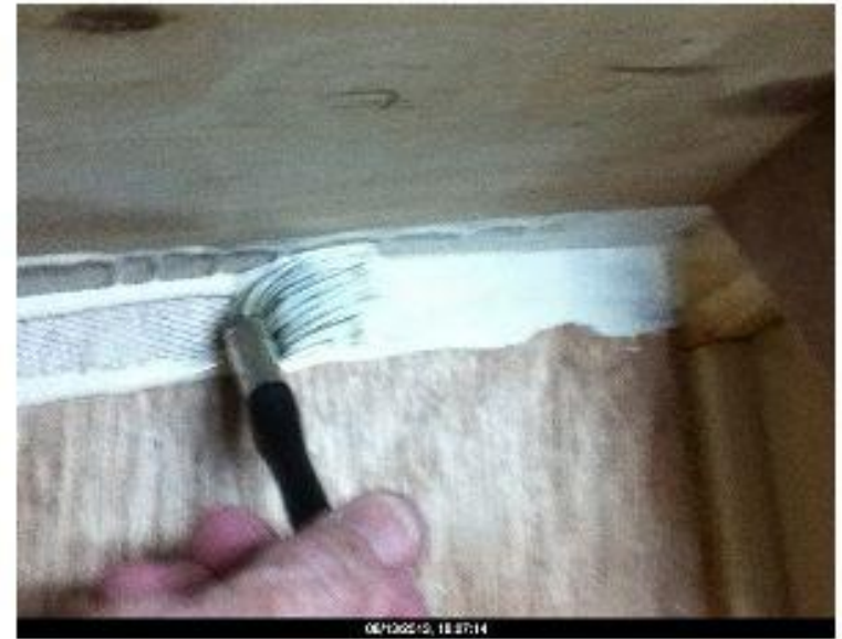
Spreading glue with a small brush
